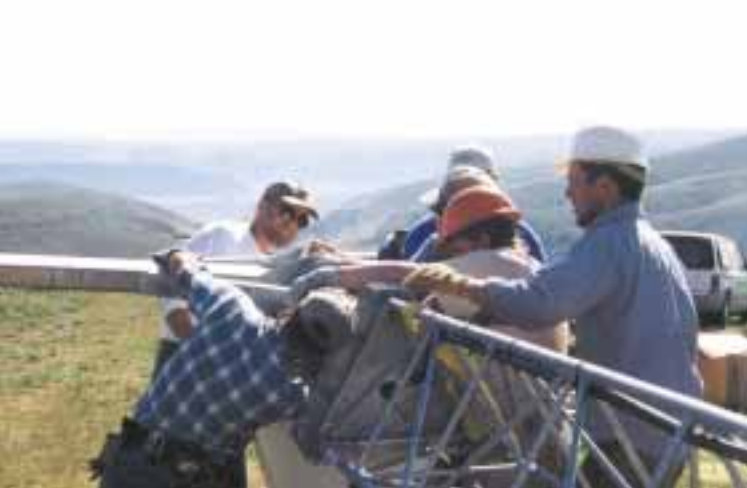
Muscling the Bergey's tail into position.
