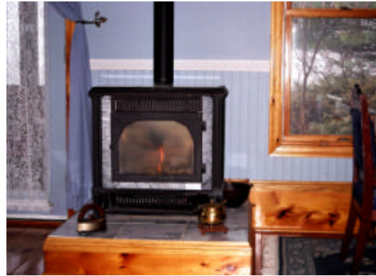
Propane fireplaces, radiant heaters and free standing units such as this model require no electricity and can be sized to meet the heating requirements of any house. They also look a lot better than the $5,000 furnace in the basement.
