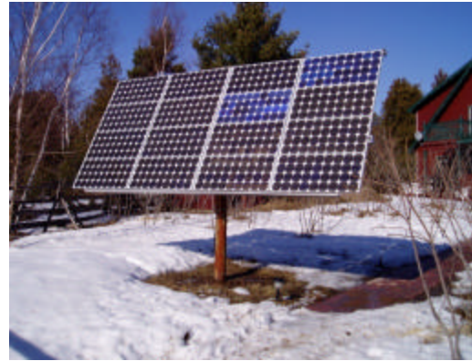
Unlike fossil fuels or nuclear energy, renewable sources are just that, renewable. No matter how much sunlight we capture with our photovoltaic panels, there will always be more for everyone else, and no dumping today's pollution on tomorrow's children. A 1200 Watt peak output PV array on a sun tracker mount.
