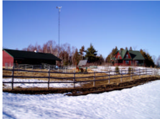
This off-grid property is typical of many rural properties, with the exception of the wind turbine, photovoltaic panel, and lack of hydro bill!
