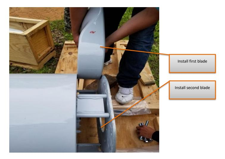
Two blades can be installed before the turbine is lifted. While the turbine is being lifted they can be rotated around for the easiest installation of the third blade.
