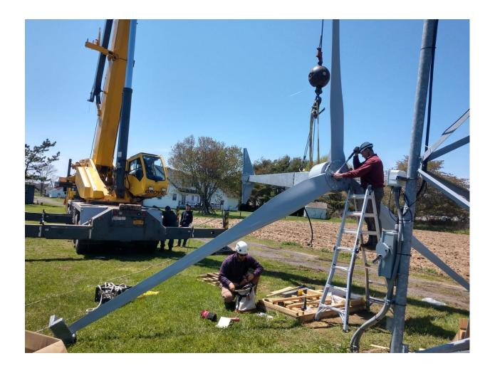
At this time the tag line should be installed to assist in raising the turbine.
