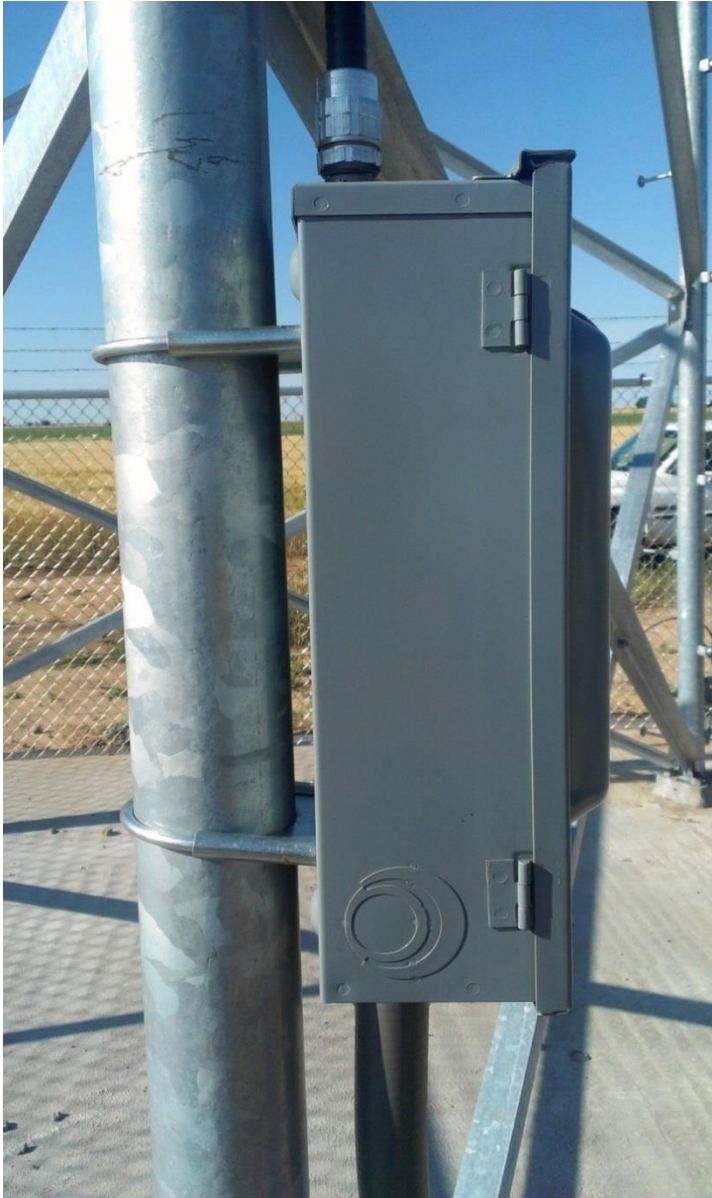
Figure 13: Attachment of Disconnect Switch
