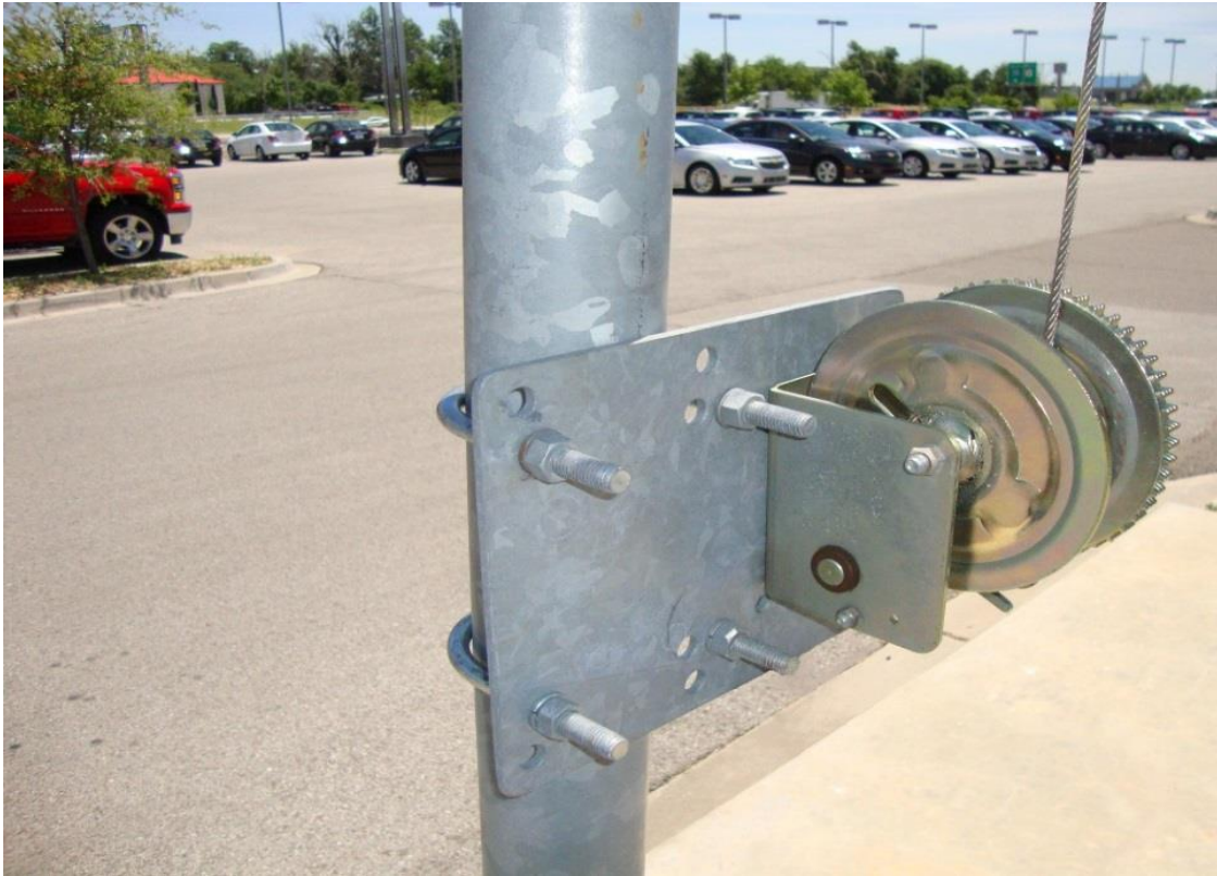
Figure 10: Winch Mounting on SSL Towers
