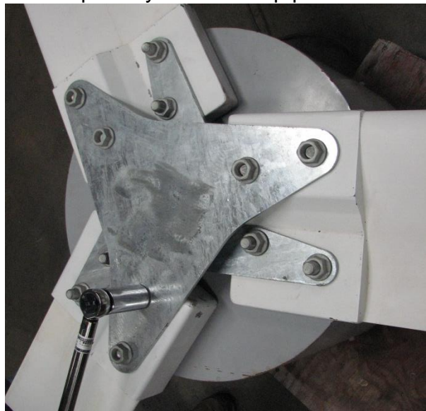
Attach primary blade-clamp plate second
