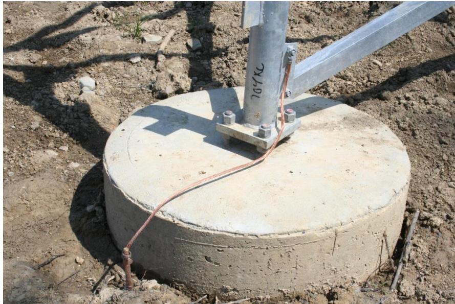
Figure 19: Tower Leg Grounding (Grout NOT Shown)
